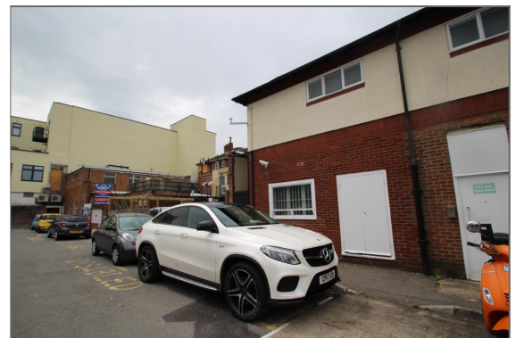
Rear access view
